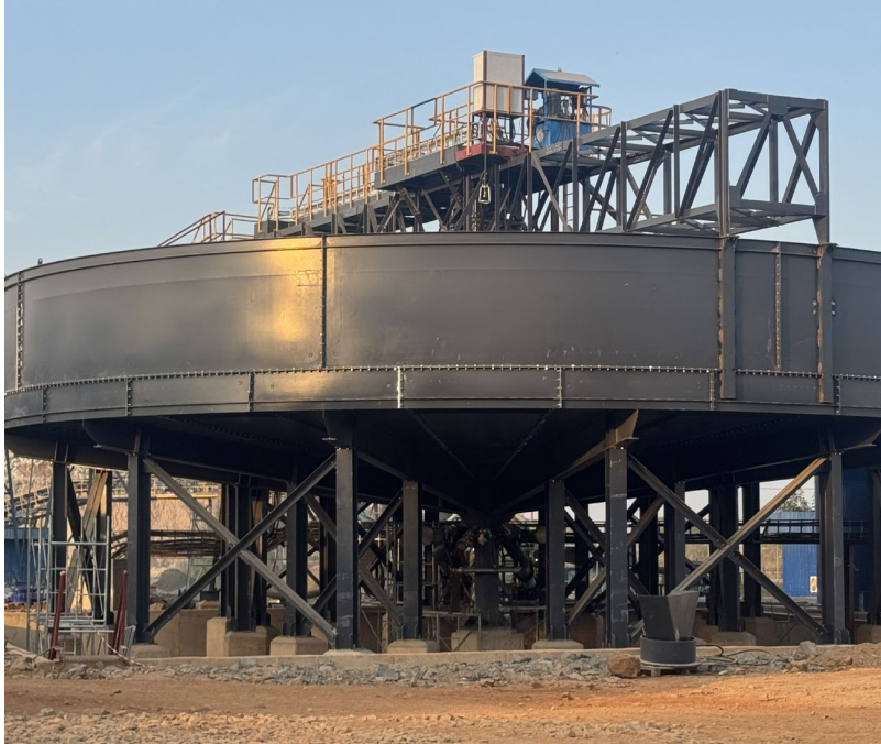
Figure 9: Installation of Pre-Leach Thickener
