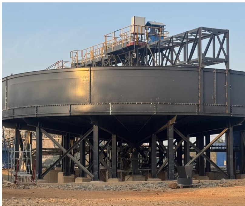
Figure 5: Installation of Pre-Leach Thickener
