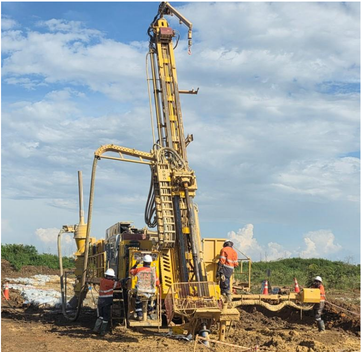
Figure 8: Reverse Circulation Drilling at Eastern Porphyry
