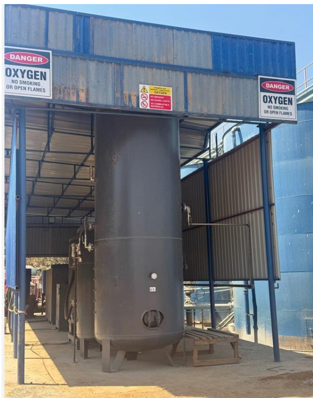
Figure 4: Installation of Oxygen Plant to Improve Slurry Oxidation
