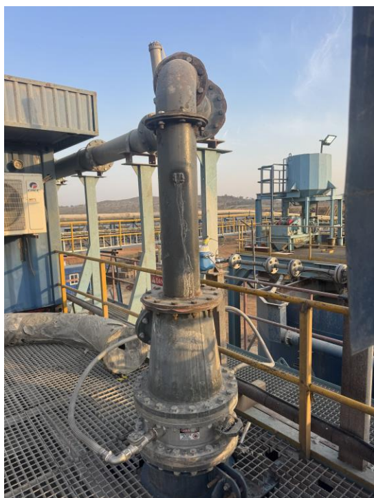
Figure 6: Aachen ® Reactor Installed and Commissioned to Improve Processing Efficiency
