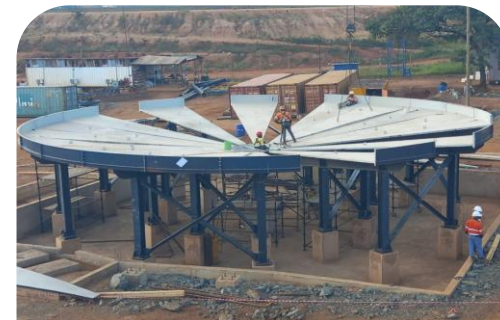
Pre-Leach Thickener Erection in Progress
