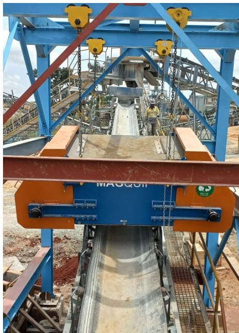
Figure 8: Installation of New Belt Magnet
