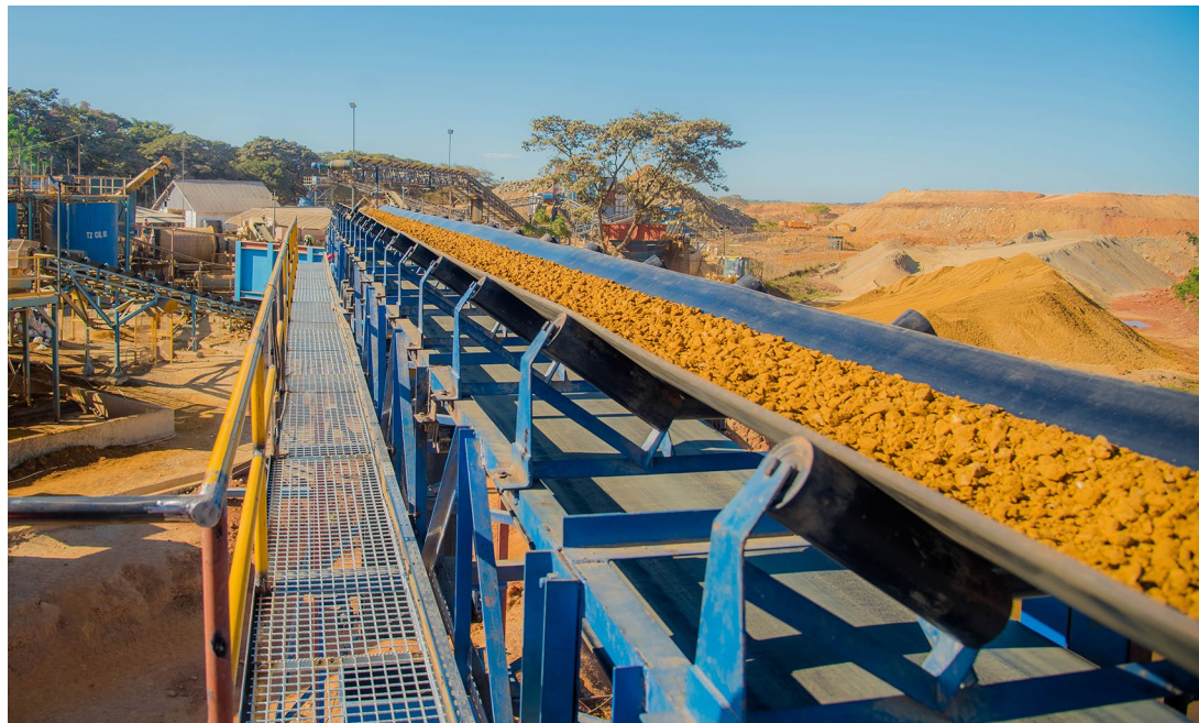
Figure 3b: Buckreef Gold Ore Moving Through Crushing Circuit
