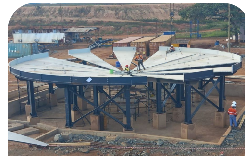
Pre-Leach Thickener Erection in Progress
