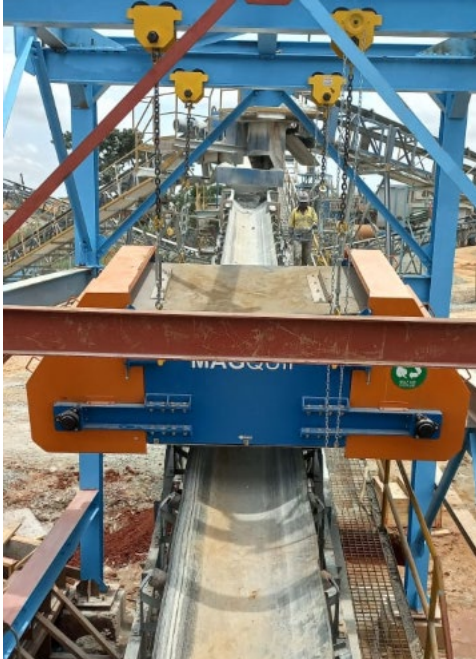
Figure 8: Installation of New Belt Magnet
