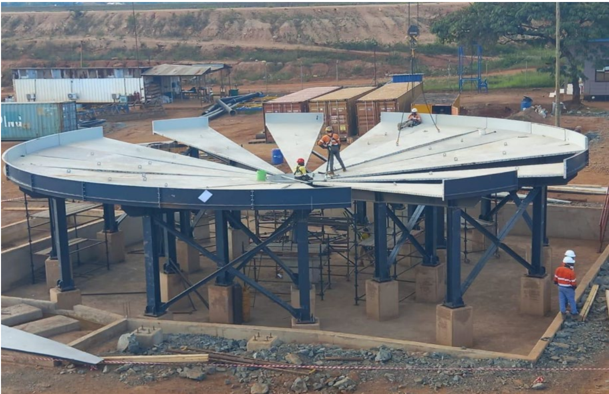
Figure 9: Pre-Leach Thickener Erection in Progress
