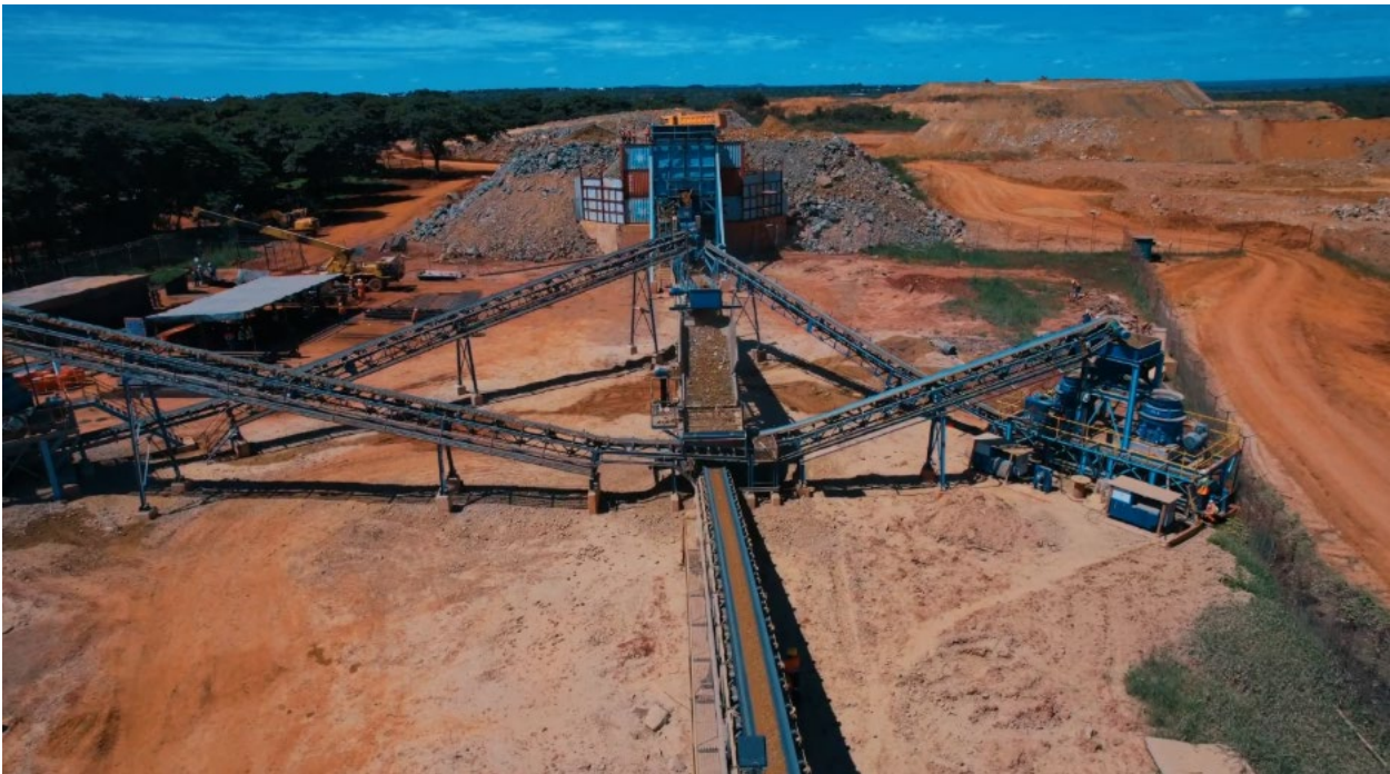
Figure 2: Buckreef Gold Crushing and Conveyor Circuit
