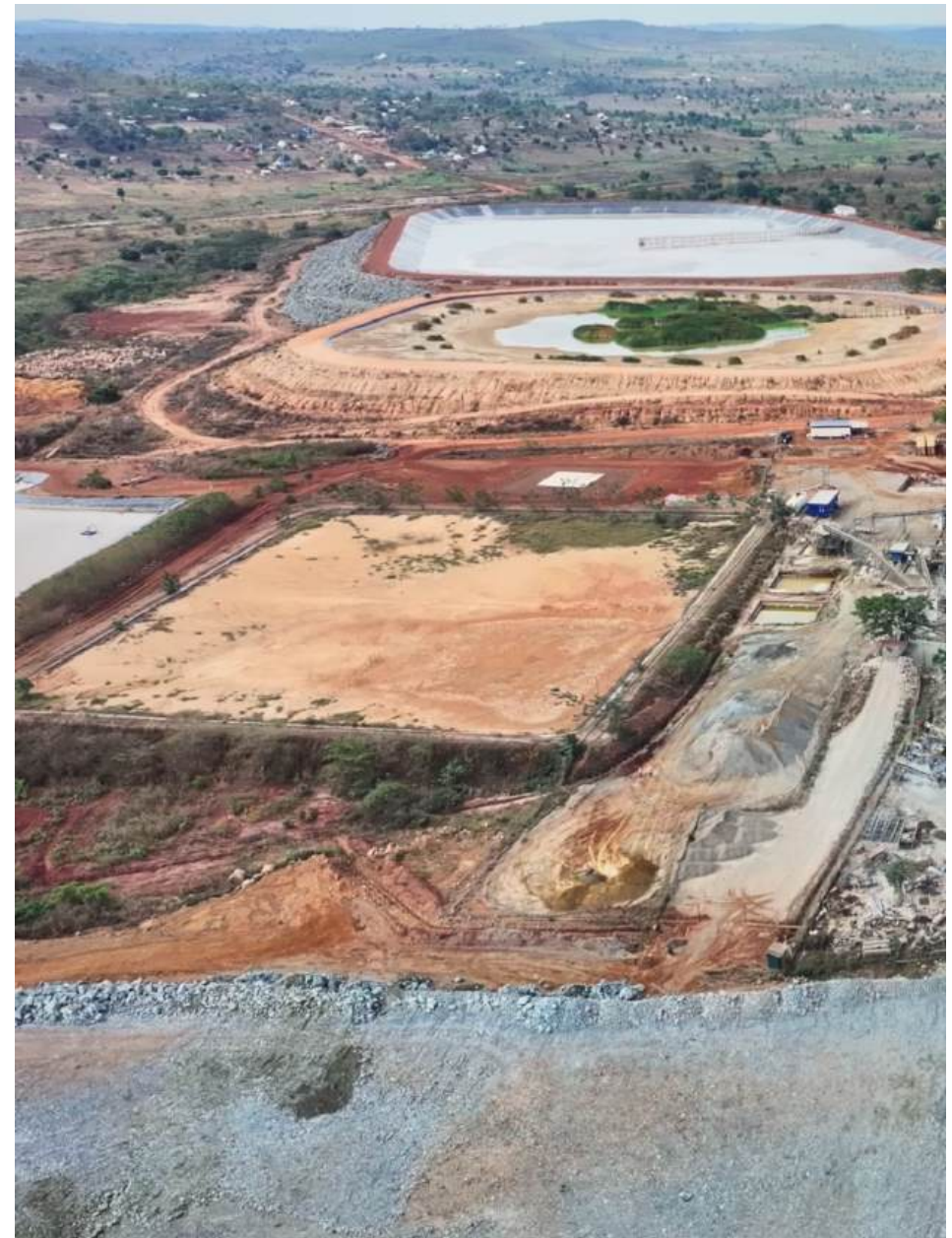
Aerial view of the tailings facilities at Buckreef operations.
