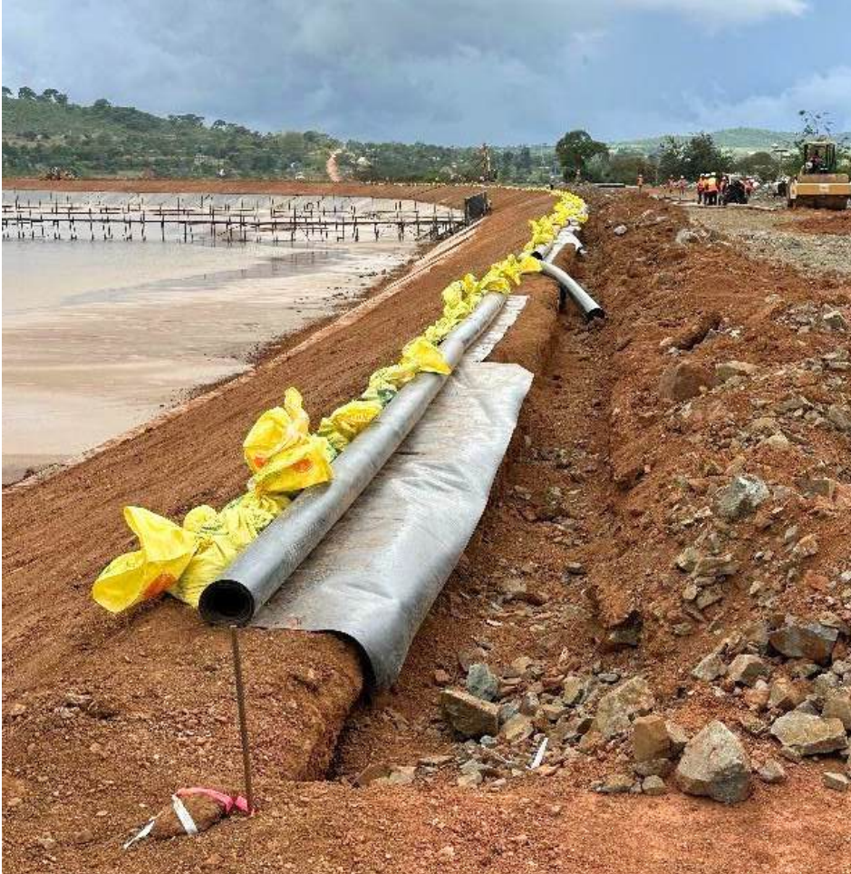
Installation of the Phase II Lift One liner at TSF 2, Cell 2
