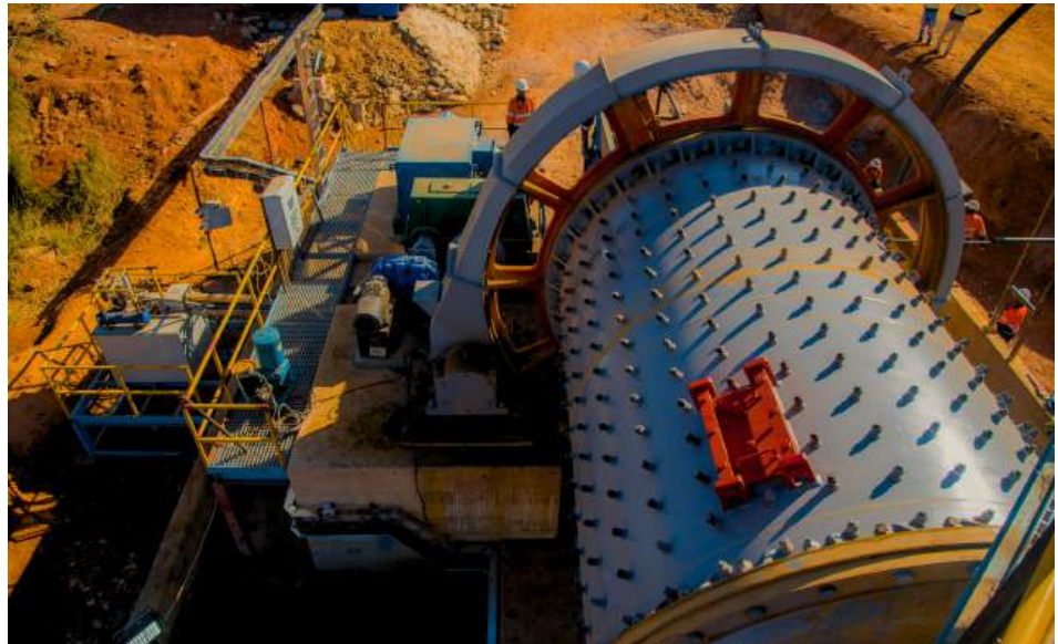
Ball mill at the Buckreef Gold processing plant
