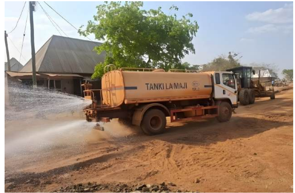
Water used for dust suppression during local community road upgrading works.
