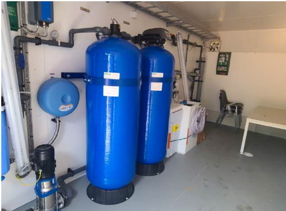
Water Treatment Plant
