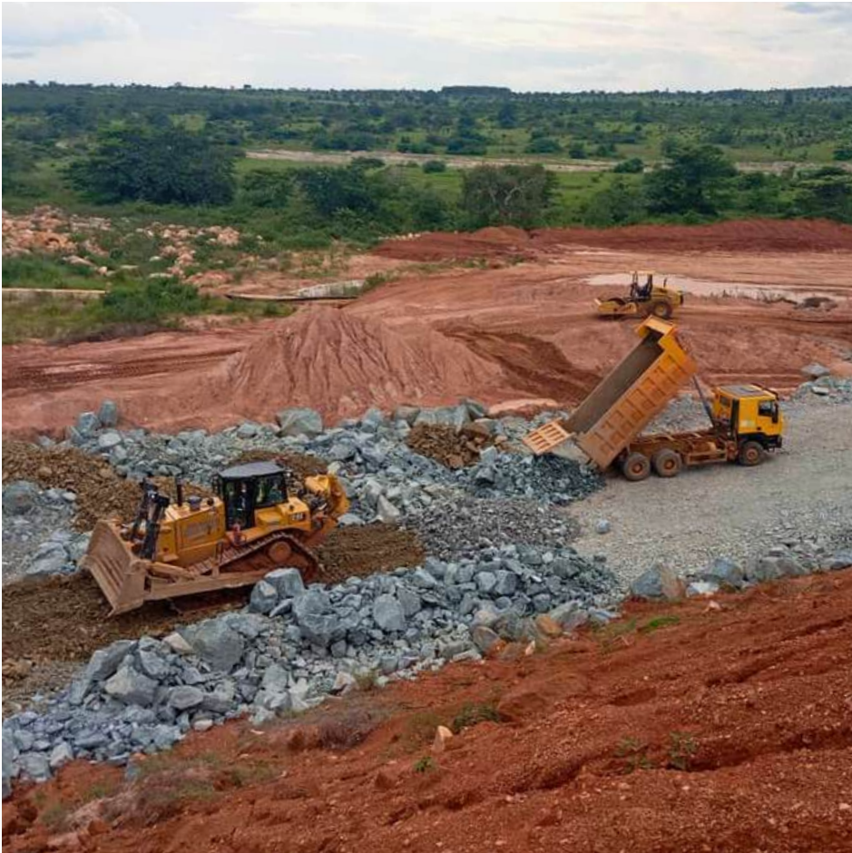
TSF 2 Cell 2 expansion earthworks at the Buckreef Gold Project.
