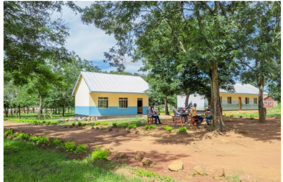
New classroom at Lubanda Primary School
