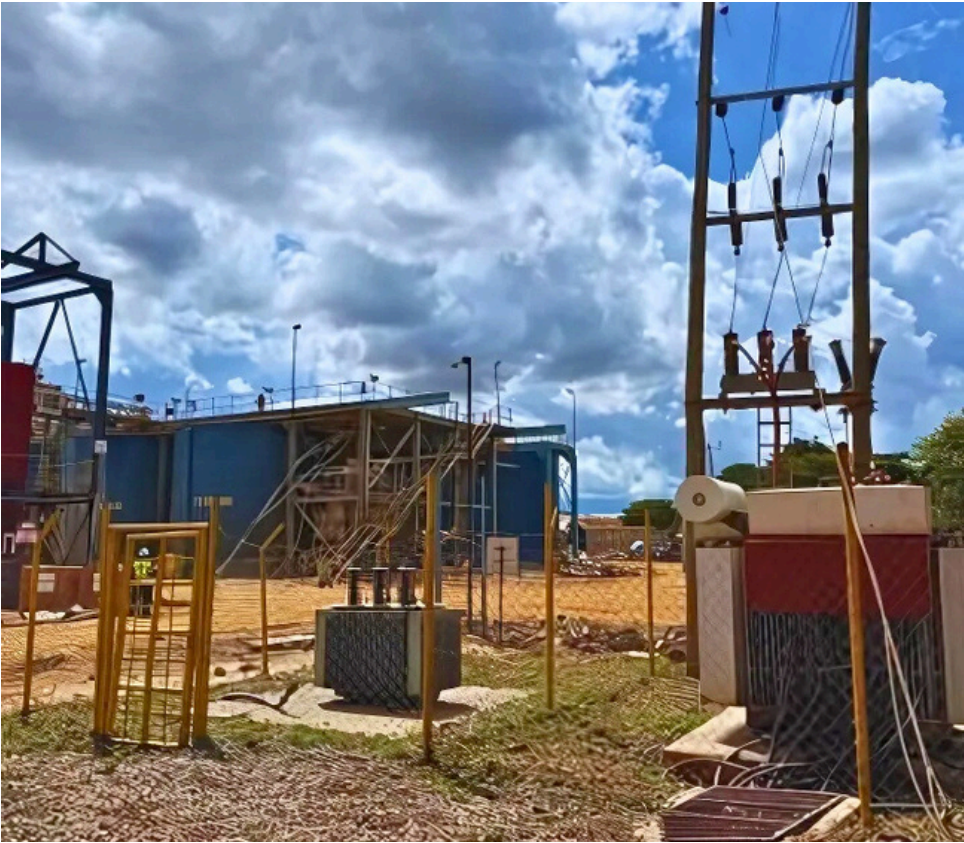
National grid TANESCO Tapping point to the process plant
